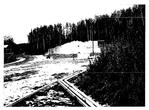
Photo 11: Tank Farm 6; Header #1 and the fuel line to Tank Farm 7 are shown in the foreground to the right. The single pipe branching to the left serves the city building and the water treatment plant. Tank Farm 6 is encompassed by a locked fence. A dispenser for local fuel consumption is located in the white shed shown above.
